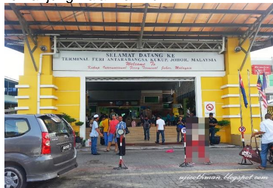
Gambar 6. Terminal Ferry Kukup , Malaysia
